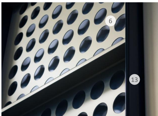
Detail Aluminium-Lochblech Detail aluminium perforated metal sheet
